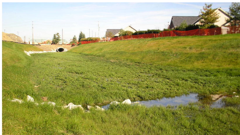
Application of over-wide channel technique. Source: EMH&T
